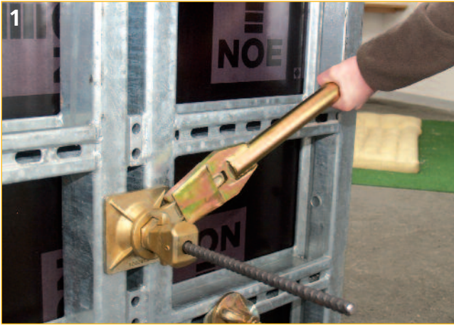
1 Open the nut with the Socket tool – careful, efficient and without noise.
