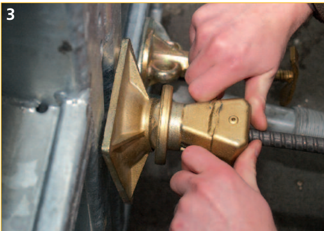
3 To unlock the enclosed 2 nut halves press the body of the rapid locking nut towards the formwork while holding back the two wings with the forefingers.
