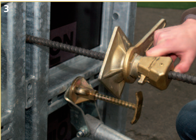
3 After placing the second side of the wall formwork simply push the rapid locking nut over the bar until the counter plate touches the formwork – no screwing necessary!
