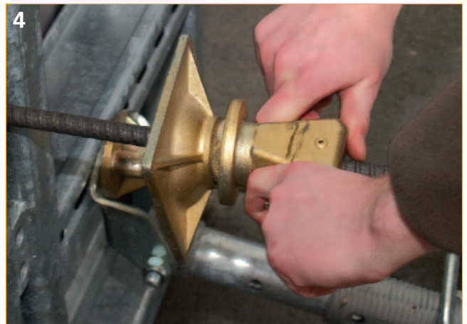
4 After that the rapid locking nut can be pushed over the bar, holding the wings simultaneously.
