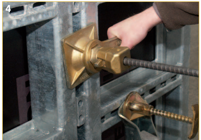
4 Press the nut easily by hand by turning the rotating wrench.
