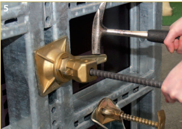
5 Simple tightening of the bar with a hammer because of the big lever arm of the wrench.
