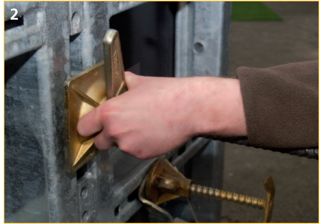
2 After releasing the tension in the bar turn the nut by hand with 2 or 3 rotations to move it a little bit apart from the formwork.
