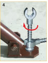
4. Final tightening of the screw by simply turning it with second scrwe-in set. Because of the form of a screw spanner of the scrwe-in set also a conical flange nut can be tightened.
