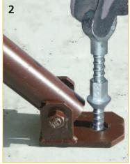
2. Screw bolt into the anchoring ground.
