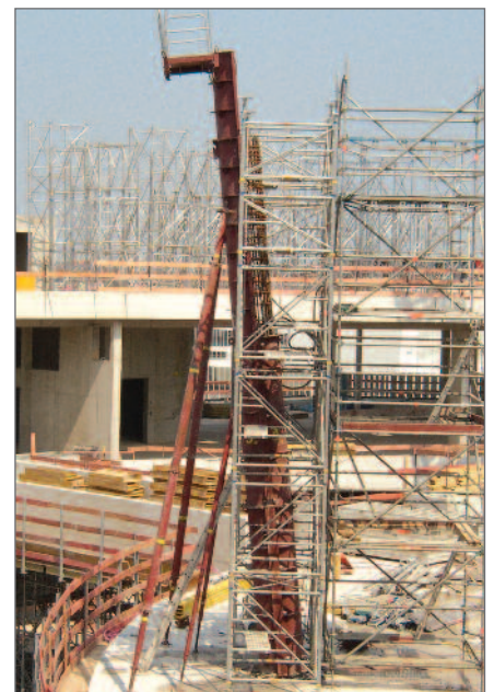
Inclined formwork Ø 800 mm with special base-element
