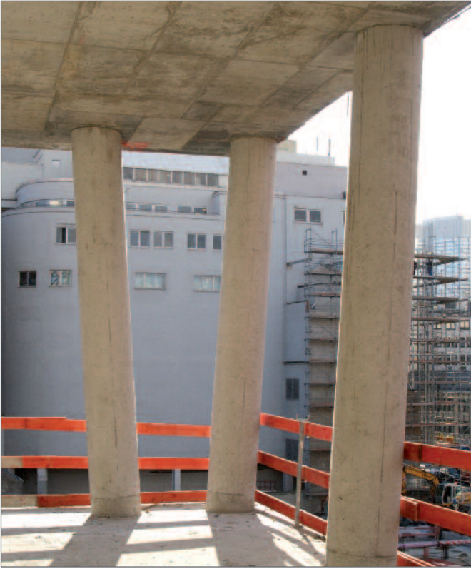
Inclined columns, poured with rental formwork and beveled special base elements
