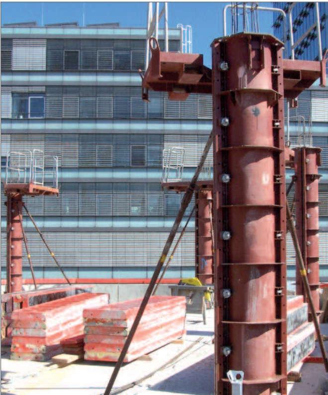
Formwork with working platform, for high safety while pouring the concrete
