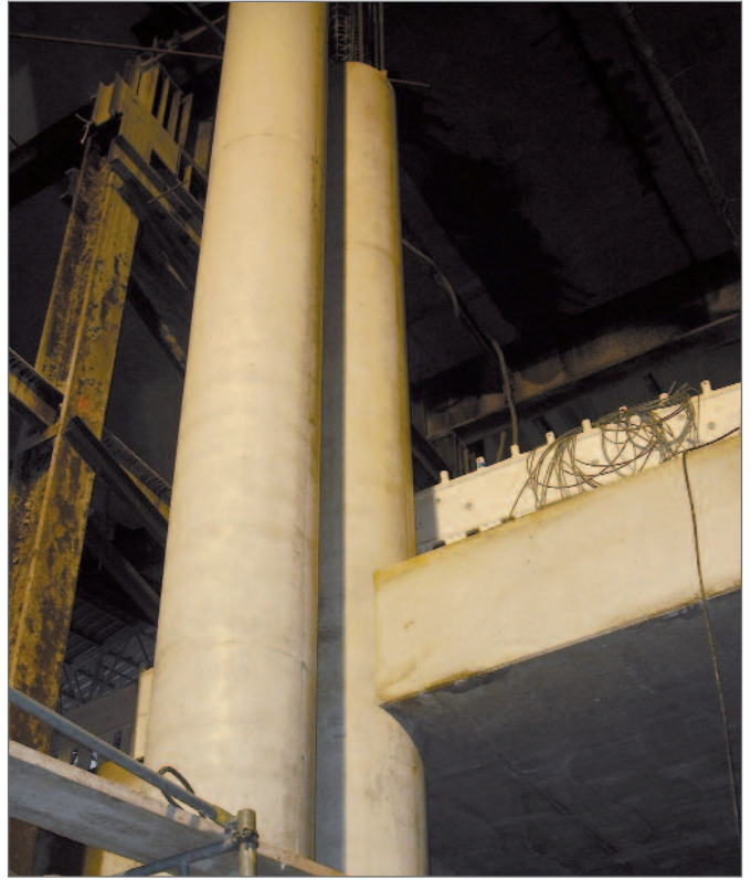
Columns in an underground train construction site. Heights up to 12 m were poured in a single operation.
