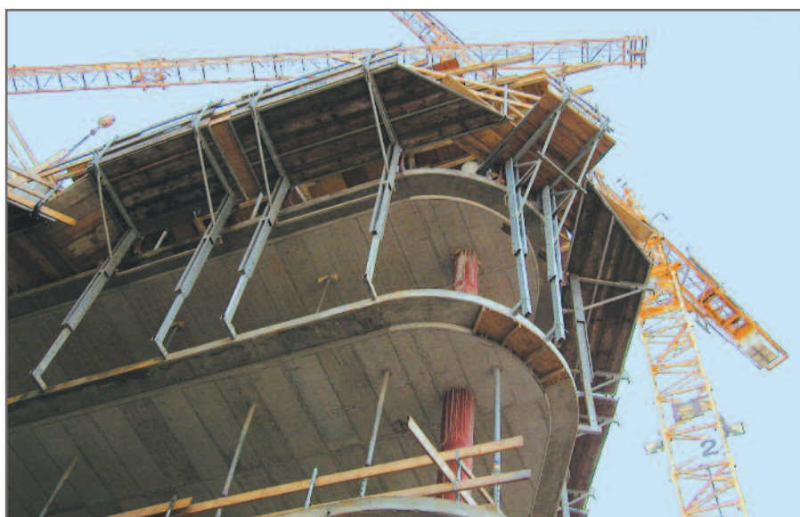
Subsequent use of the working platforms for reorganization purposes with mounted front scaffolding, free passing of vehicles during stage of working.
