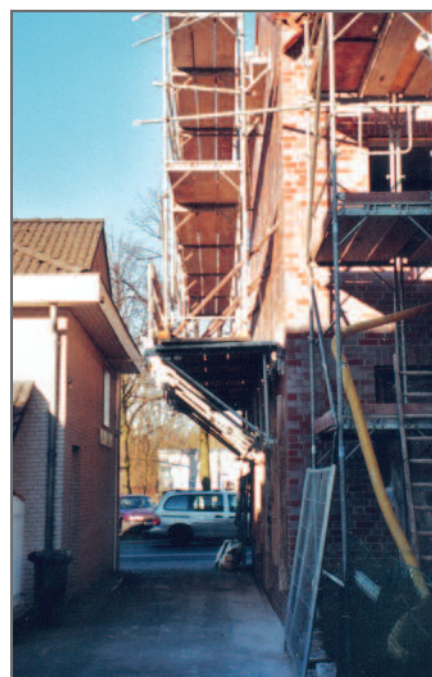
Subsequent use of the working platforms for reorganization purposes with mounted front scaffolding, free passing of vehicles during stage of working.
