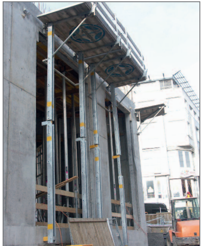
Extension girder, connected, for bridging from up to 6 m window openings
