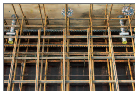
Installation-kits nailed to the shuttering of the slab
