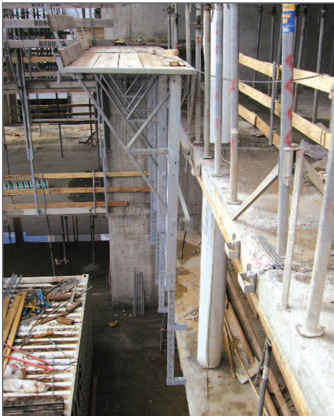
Foldable working platform with long base frame and extension girders at pier façades, suspended one meter above floor level.
