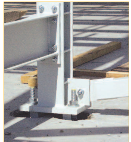
Exact mounting with fitting installation template
