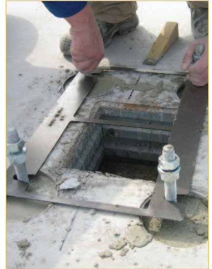
Exact mounting with fitting installation template
