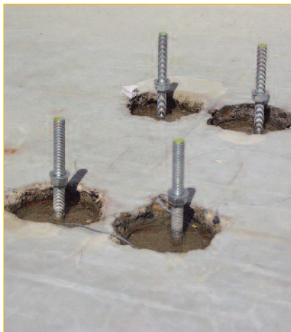
Pouring the grout into the tubes
