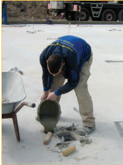
Pouring the grout into the tubes
