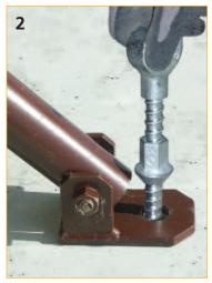
2. Screw bolt into the anchoring ground.
