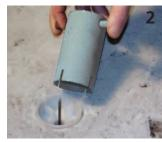
Removing of clamping flange with removing tool
